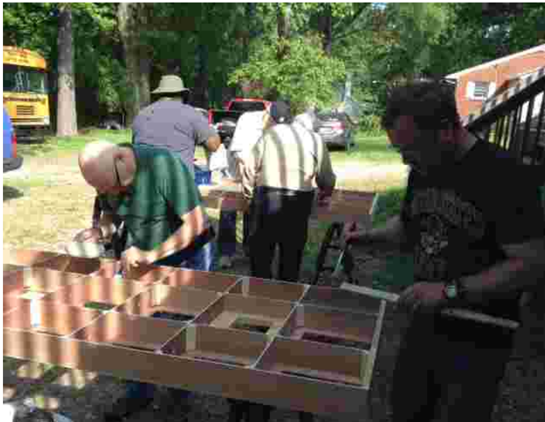
Working on the new HO modules at Bill Swint's house.
